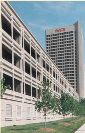
Coca-Cola Parking Structure Atlanta
