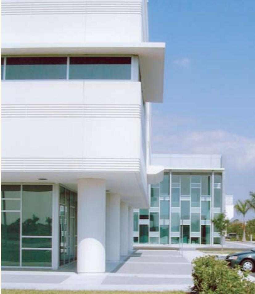
**Fig. 7 High-reflecting (usually light-colored) surfaces help mitigate urban heat islands.**
