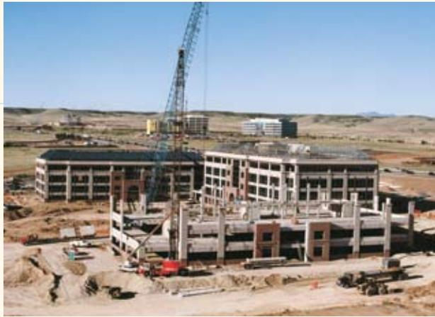
**Fig. 3.** All three total precast concrete buildings are LEED certified. CH2M Hill World Headquarters, Englewood, CO
