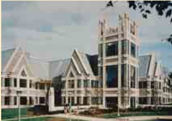
German limestone is anchored to precast panels on the Terry Sanford Institute of Public Policy at Duke University in Durham, N.C. (Architect: Architectural Resources Cambridge Inc.)
